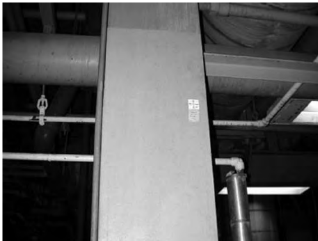
FIGURE 16.52 Adhesive-backed target attached to I-beam.
