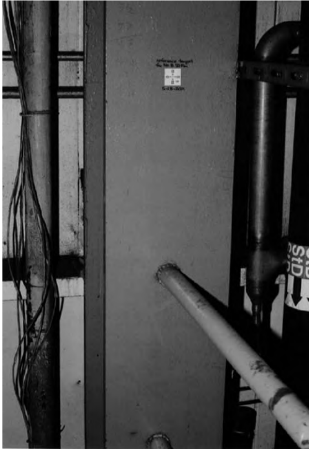
FIGURE 16.51 Adhesive-backed target attached to I-beam.
