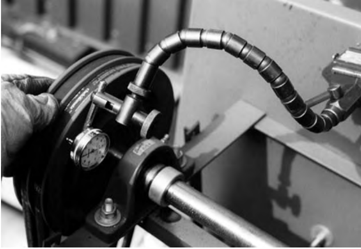
FIGURE 18.15 Face runout check on sheave.
