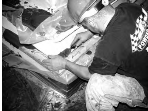
FIGURE 3.56 Scraping off the excess grout while still in the putty stage.
