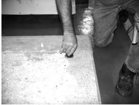
FIGURE 3.31 Neoprene sleeve to protect threads on anchor bolt.
