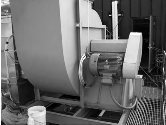
FIGURE 21.46 Belt-driven fan.
