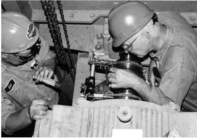
FIGURE 21.48 Aligning a direct-driven fan.
