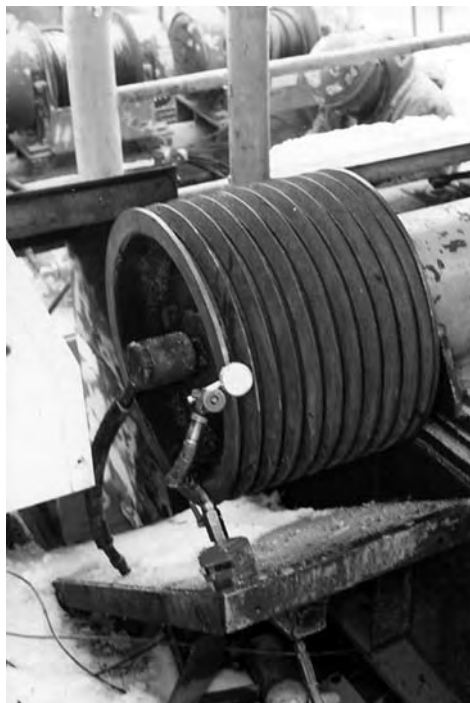
FIGURE 5.31 Measuring radial runout on a multi-V sheave.
