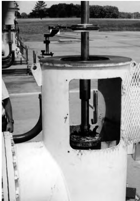
FIGURE 21.44 Checking for perpendicularity on the flange surface.
