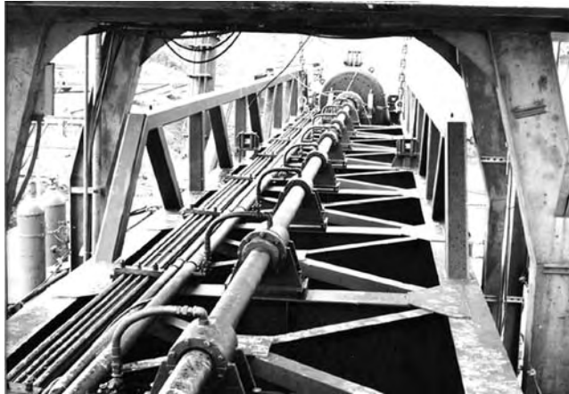
FIGURE 3.11 Series of water bearings held in place on a dredge frame.
