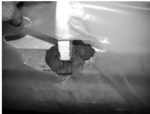
FIGURE 3.51 Plugging the leak with duct sealant.
