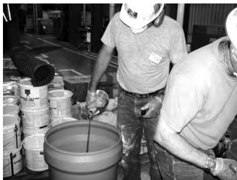
FIGURE 3.47 Mixing the grout contents.
