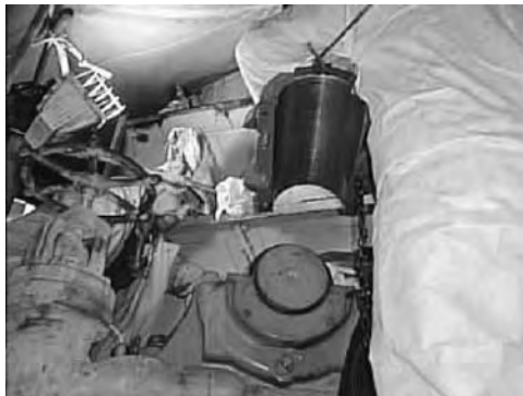
FIGURE 5.8 Checking contact on a sliding bearing with bluing.
