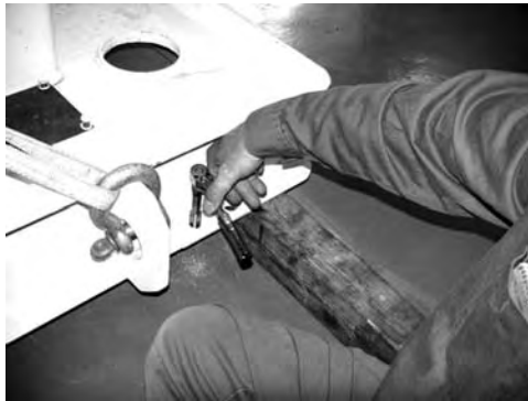
FIGURE 3.37 Cleaning the threads of the jackscrews.
