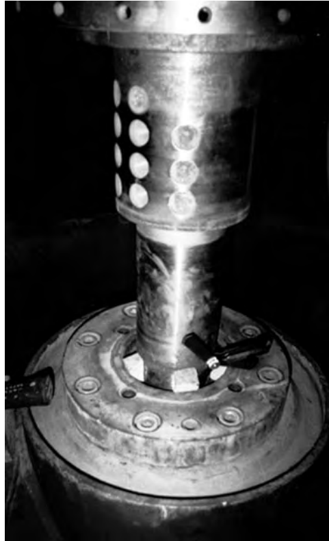
FIGURE 21.22 Wooden wedges were used to keep the pump shaft centered.
