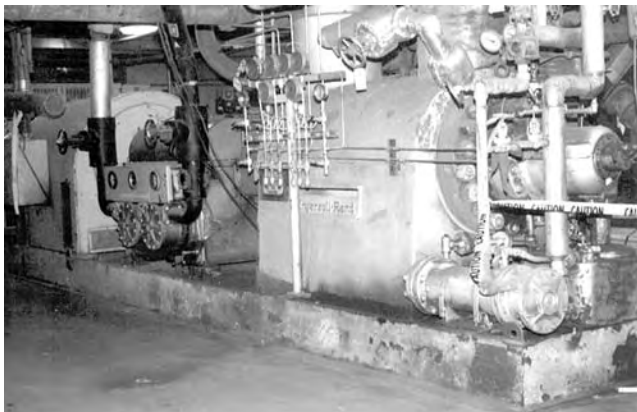
FIGURE 21.79 Motor, fluid drive, pump drive arrangement.
