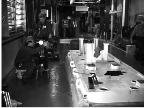
FIGURE 3.42 Double checking elevations with two independent observers.
