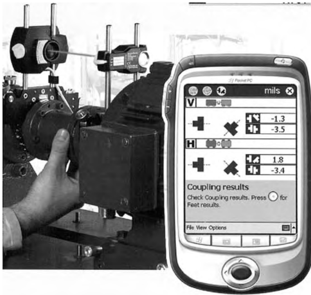
FIGURE 15.14 Pocketalign system. (Courtesy of Prüftechnik, Ismaning, Germany. With permission.)
