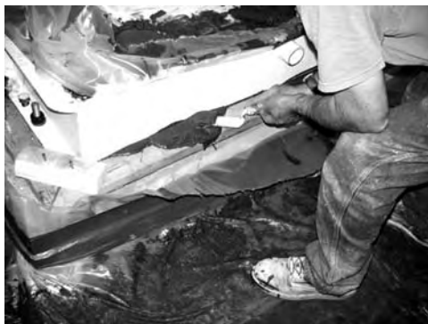
FIGURE 3.55 Scraping off the excess grout while still in the putty stage.
