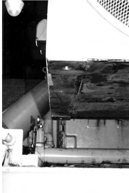
FIGURE 5.43 Cleaning the underside of the feet on a motor.
