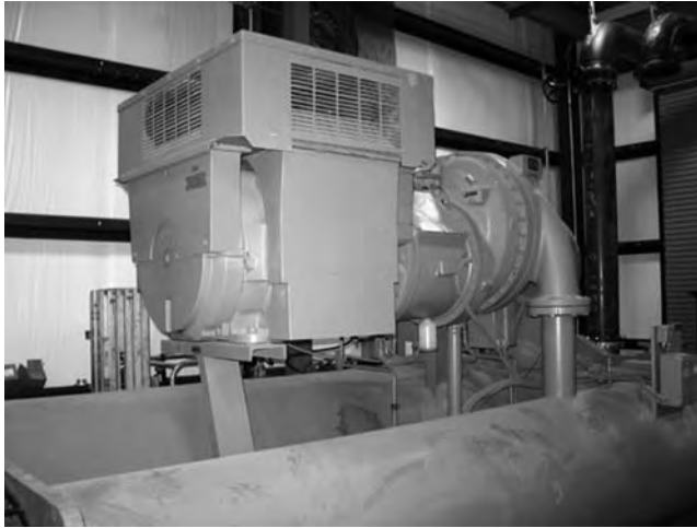
FIGURE 21.56 Chiller compressor.
