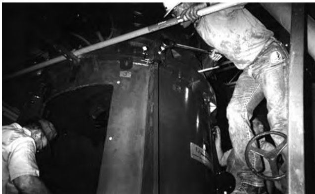
FIGURE 21.31 Adjusting the jackscrews to correct the offset misalignment.
