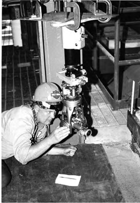
FIGURE 3.8 Optical jig transit being used to level a soleplate.
