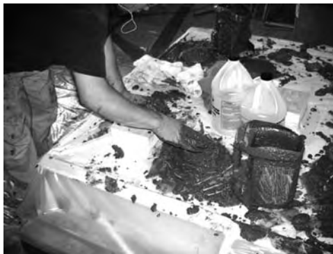
FIGURE 3.54 Hand packing the grout.
