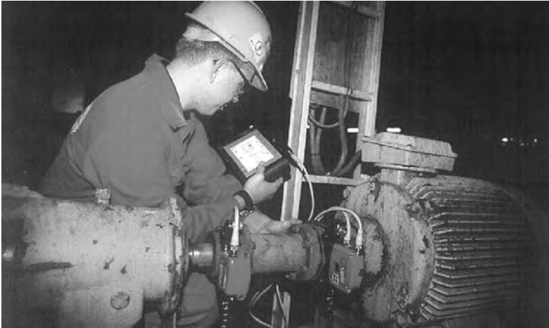
FIGURE 15.9 Shaft 30 system. (Courtesy of FixturLaser, Molndal, Sweden. With permission.)
