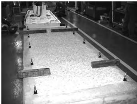
FIGURE 3.33 Ready to set baseplate onto concrete foundation.
